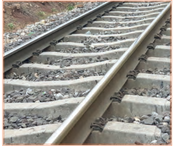
Görsel 3.17: Beton travers
